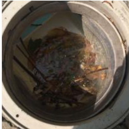
Figure 3:Dirty Pool strainer.
